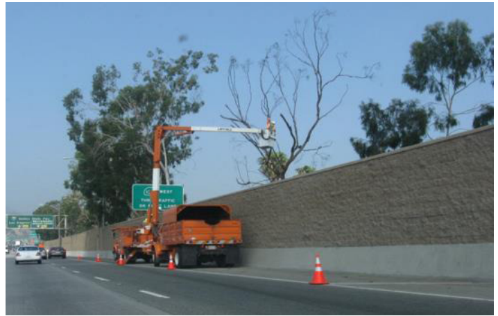
Traffic cones establish a drop zone.
